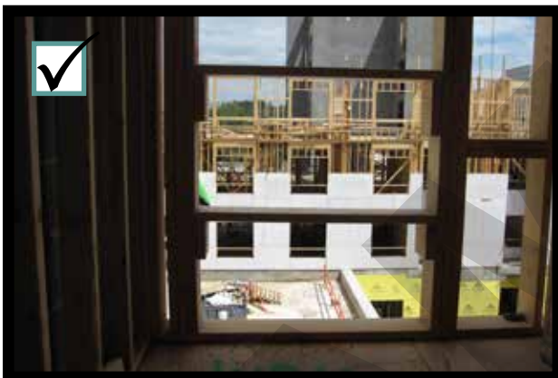
Erect guardrails around window and door openings.
