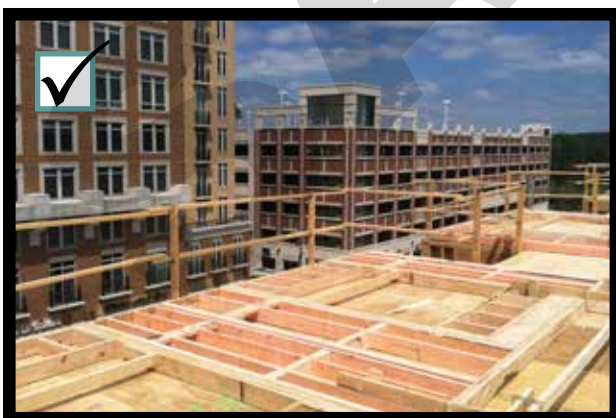
Erect guardrails around the leading edge.
